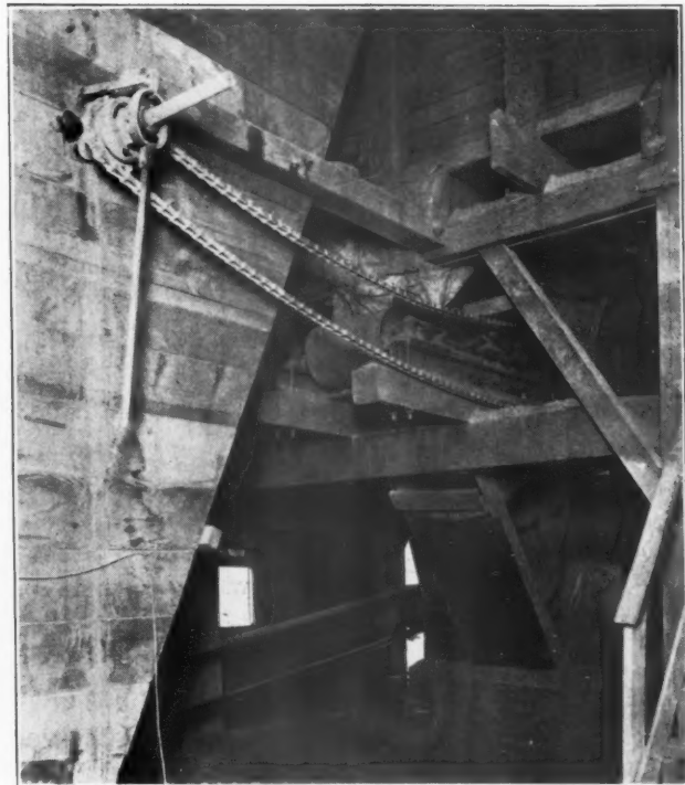
Inside View Showing Magnetic Pulley
